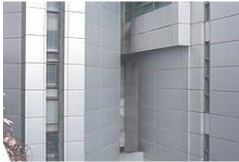
Steel building with aluminum panel frame, in Korea
