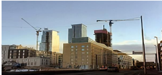
Skyscrapers under construction in Kalasatama, Helsinki, Finland (2021)
