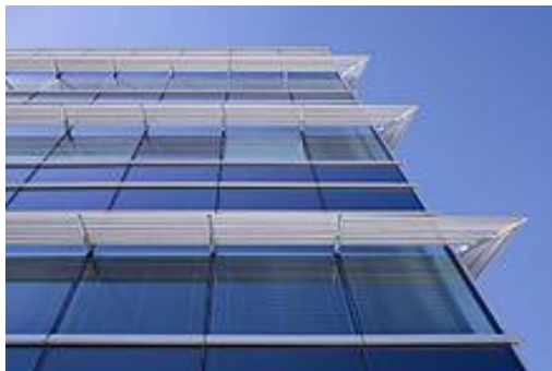
Outdoor Light Racks - Green Office Building, Denver, Colorado
