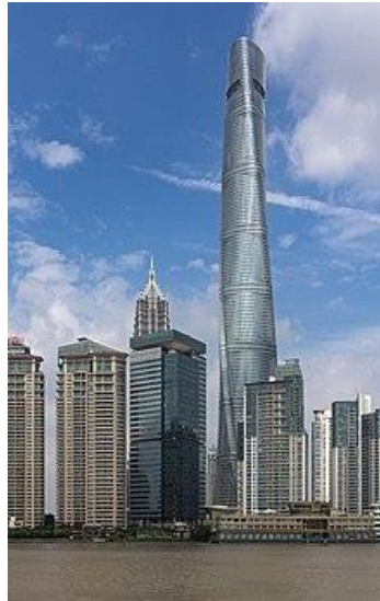
Shanghai Tower, the tallest and largest LEED Platinum certified building in the world since 2015
