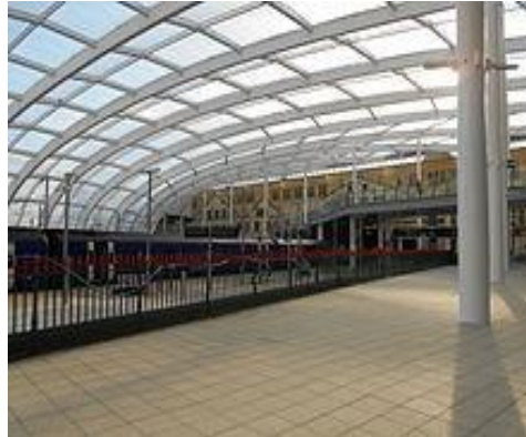
Steel frame roof at Manchester Victoria Station
