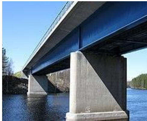
A metal beam under a bridge
