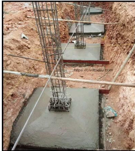
Image of isolated shallow foundation
