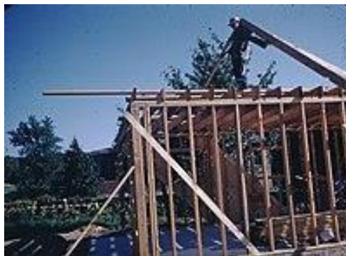
A roof shuttering in the United States around 1955
