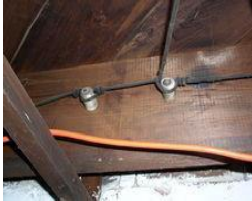
Handle and tube wiring (the orange cable is an unrelated connection wire)
