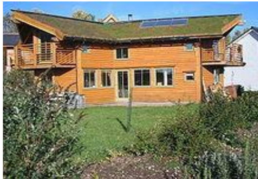
An ecological house in the village of Findhorn with a grass roof and solar panels
