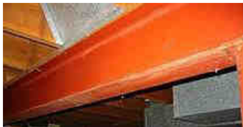
A metal I-beam used in this case to support wooden beams in the house.
