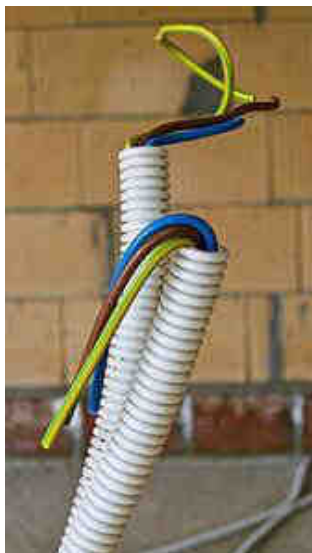
Colored wires in a flexible plastic electrical conduit commonly found in modern European homes
