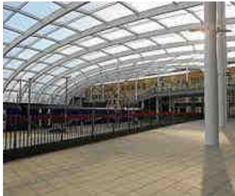
Steel frame roof at Manchester Victoria Station
