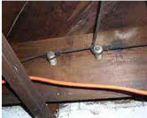
Handle and tube wiring (the orange cable is an unrelated connection wire)
